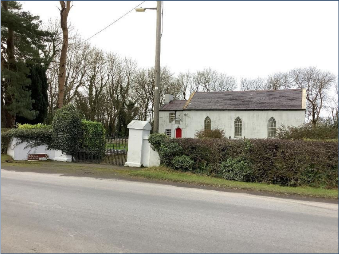
Plate 13.63: Mullafary Presbyterian Church NIAH 31302206 located to N of cable route, looking N
