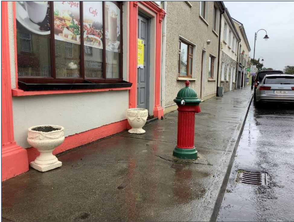
Plate 13.83: Water pump NIAH 31302603 located along TDR on Main Street Bangor.
