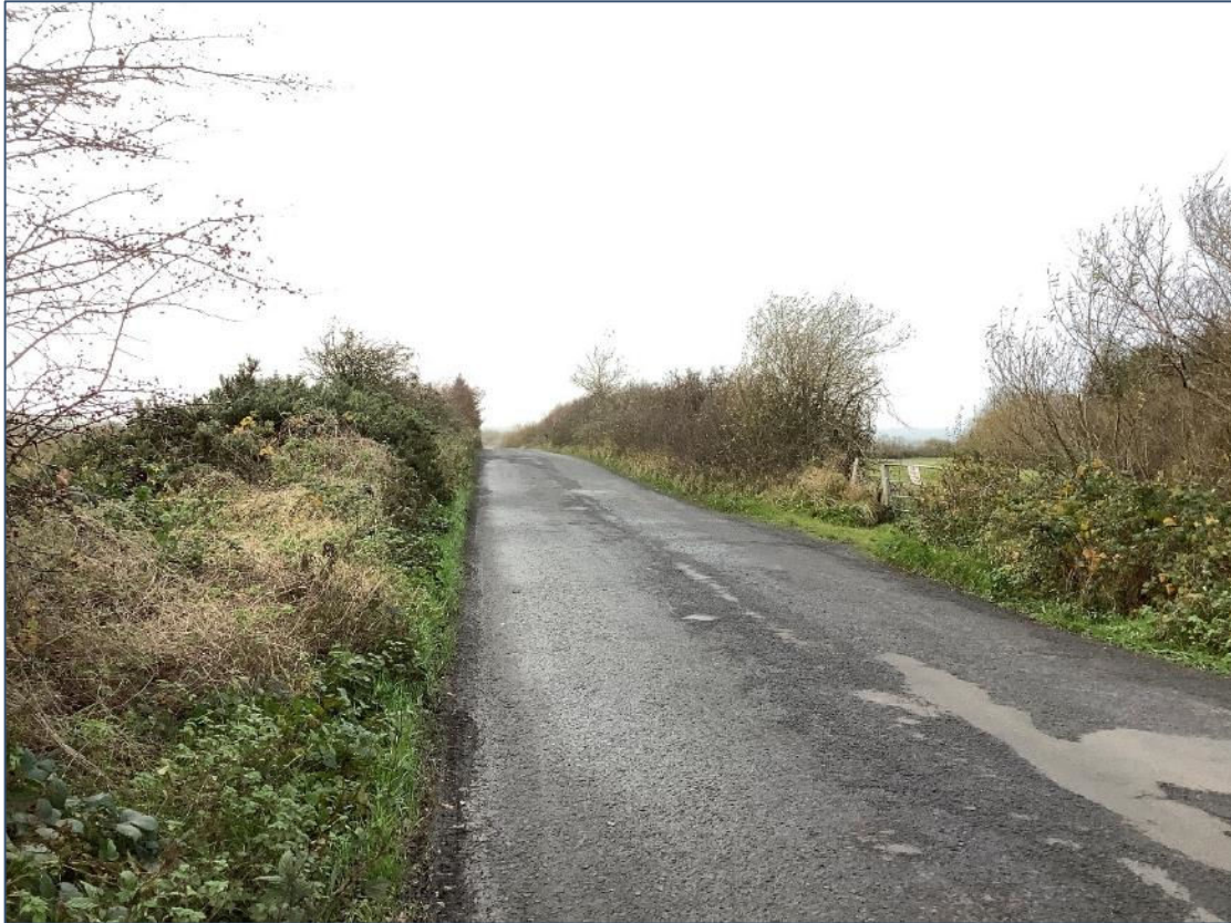
Plate 13.59: Continuation of proposed grid connection route further south looking N.
