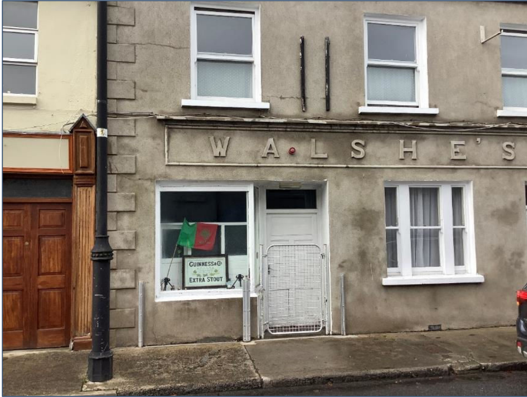
Plate 13.87: NIAH 31205006 at Church Street Crossmolina along TDR.
