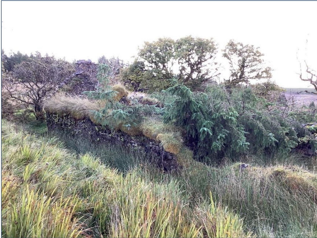
Plate 13.45: Derelict mid-late 19 th century stone building 180m to the SE of T21 at ITM E505889, N833391
