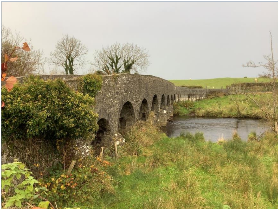
Plate 13.58: Tonrehown Bridge at Ballinagavna, /Lecarrowanteean Tds along cable route.
