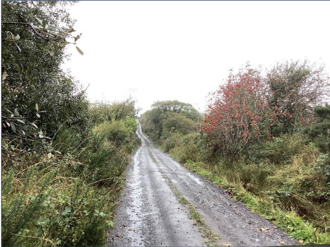
Plate 13.51: Grid connection cable route looking NE.
