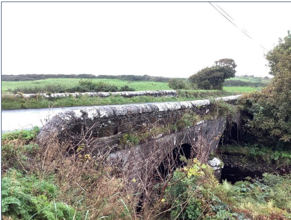
Plate 13.78: Killerduff Bridge along the TDR, NIAH 31300704
