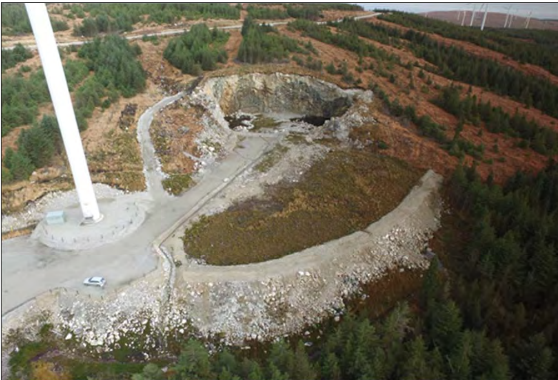
Plate 1: Borrow Pit prior to backfilling (c.2016).
