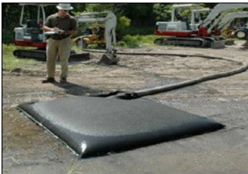
Plate 2-1 Silt Bag under inspection
