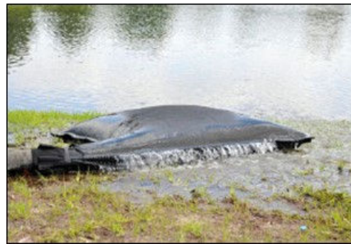
Plate 2-2 Silt Bag with water being pumped through
