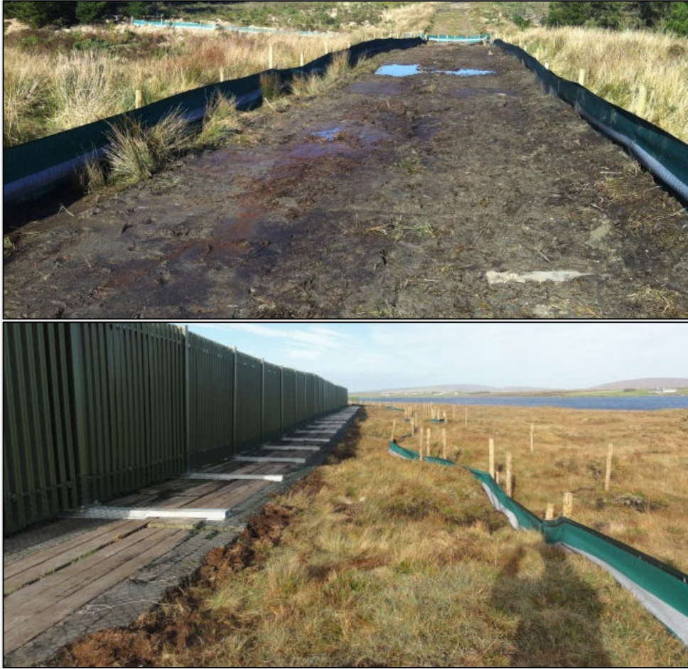
Plate 2-4 Typical Silt Fence Details
