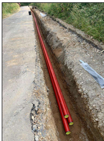
Figure 2 - Typical 110kV Underground Duct Installation
