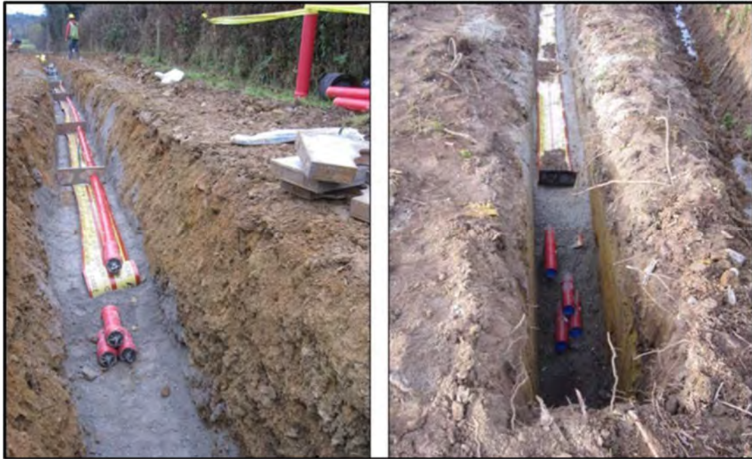
Plate 4-7 Standard Cable Trench View
