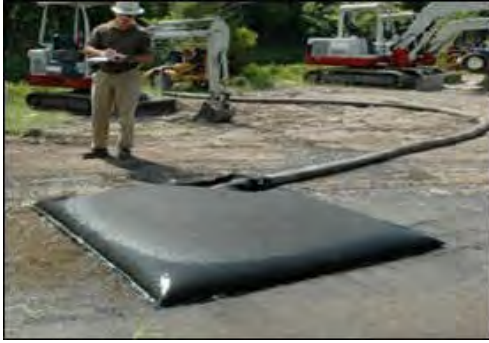
Plate 4-3 Silt Bag with water being pumped through
