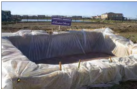
Plate 4-3 Concrete washout area
