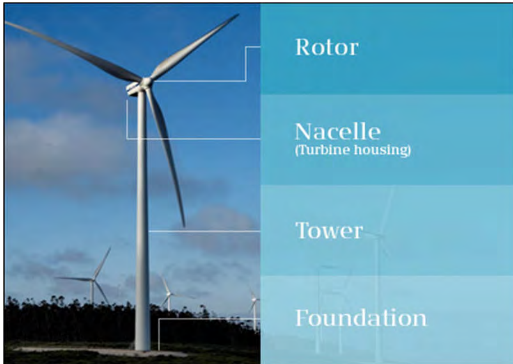
Plate 4-1 Wind turbine components
