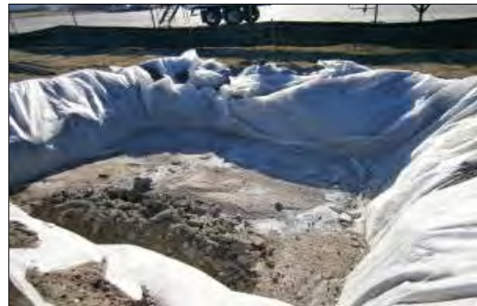
Plate 4-4 Concrete washout area
