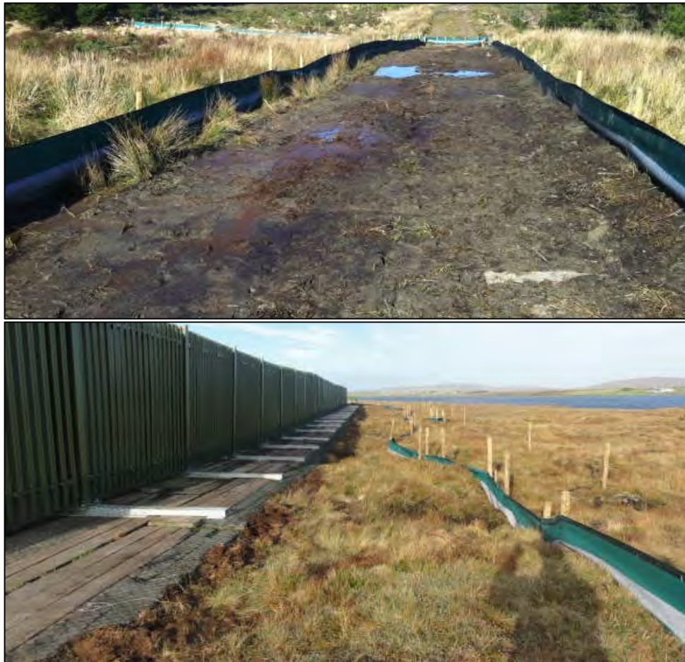
Plate 4-6 Silt Fence Details
