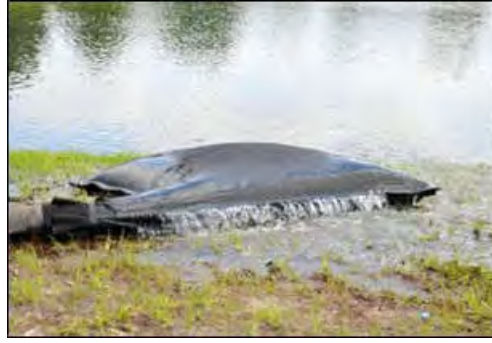
Plate 4-4 Silt bag under inspection
