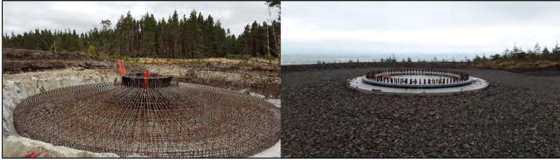
Plate 4-2 Turbine 'Anchor Cage' and finished turbine base
