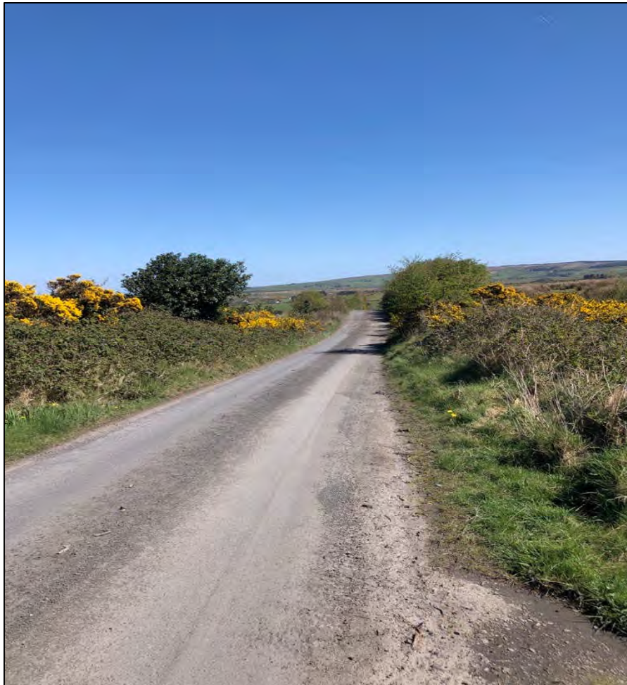
Plate 6-16 Existing Road (BL3) into which the cable is going to be laid.
