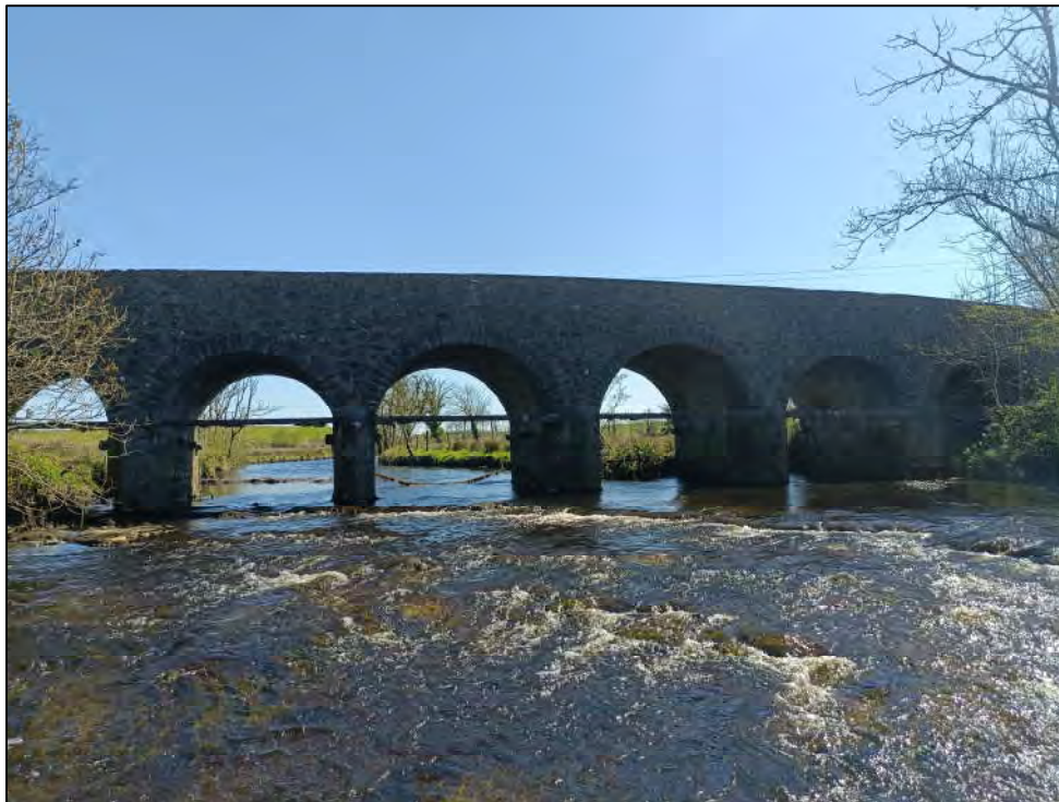
Plate 6-17. Cloonaghmore River along the Grid connection route
