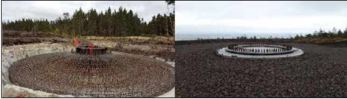
Plate 2-1 Turbine 'Anchor Cage' and Finished Turbine Base
