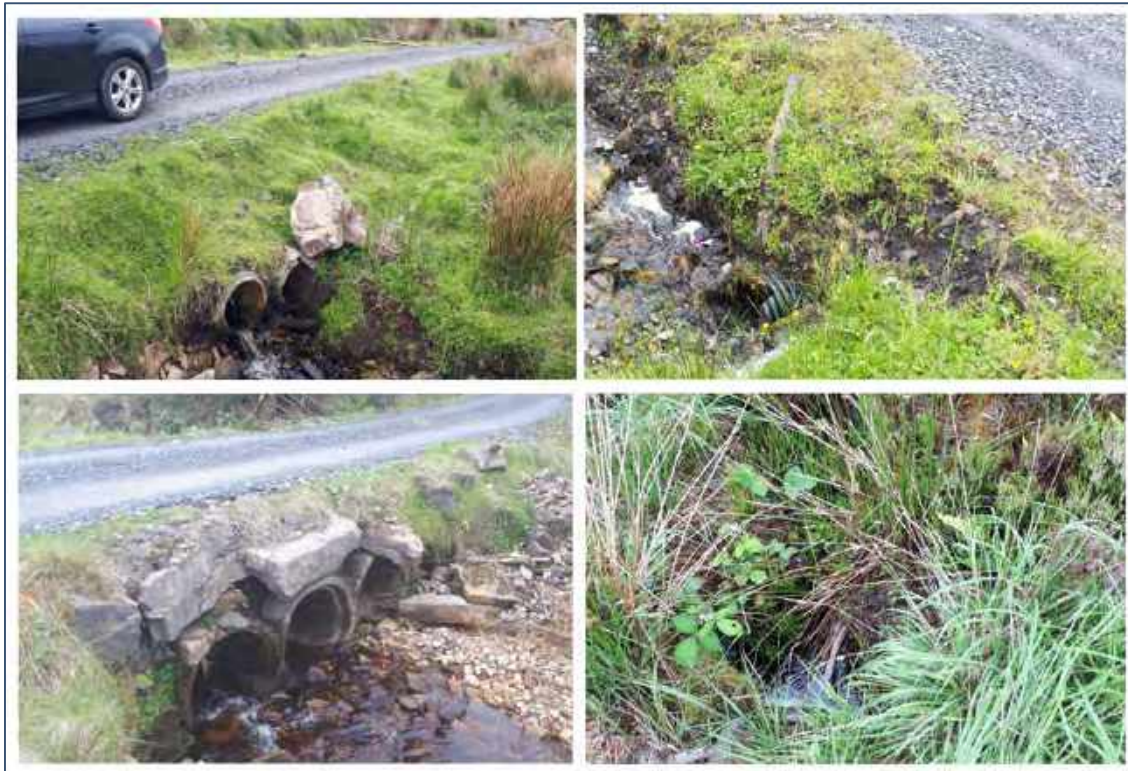
Photo 3: Examples of Pipe Culverts (Source, FT)
