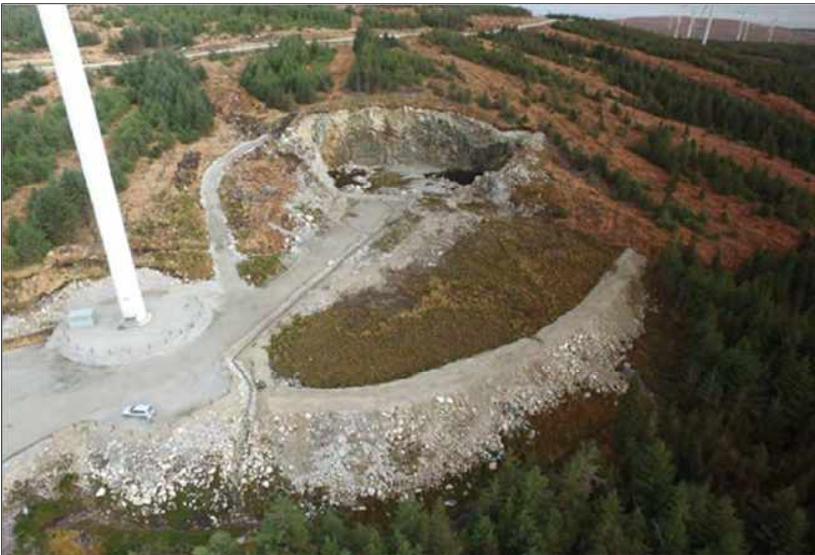
Plate 1: Borrow Pit prior to backfilling (c.2016).
