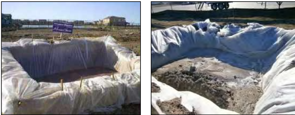
Plate 6-1 Typical concrete shoot wash out areas
