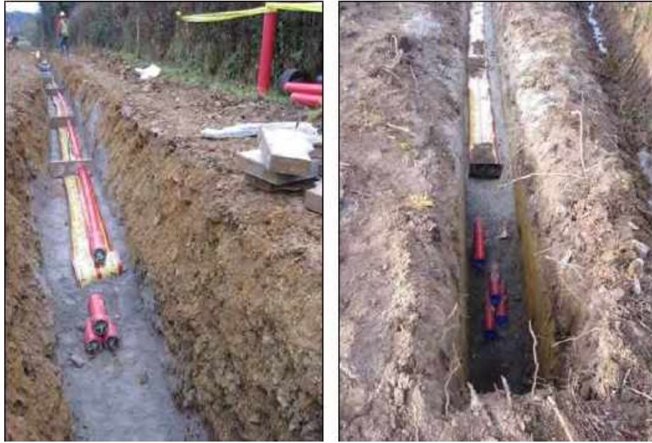
Plate 2-1 Cable Trench View
