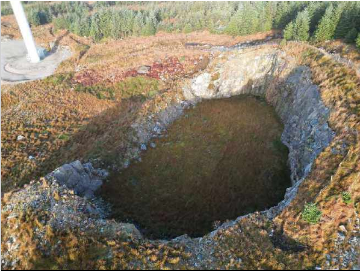
Plate 2: Borrow Pit following backfilling (image taken in 2023).
