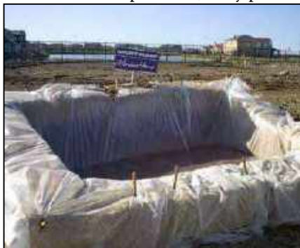
Plate 3-1 Typical concrete shoot wash out areas
